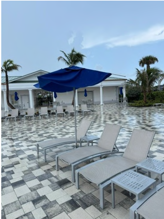
Storm-damaged pool deck umbrella
