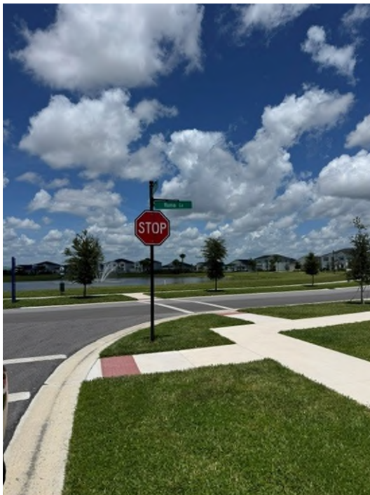
Missing street-name panel / hardware issue
